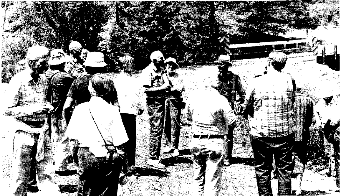
Wayne conducting a "Botany 1A Class" in the wide place on the road near Whiskey Creek. Whiskey Creek bridge is in the background.
